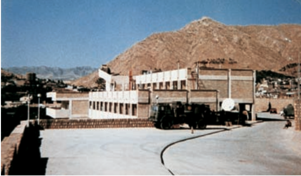
Communications site at Dahuk
